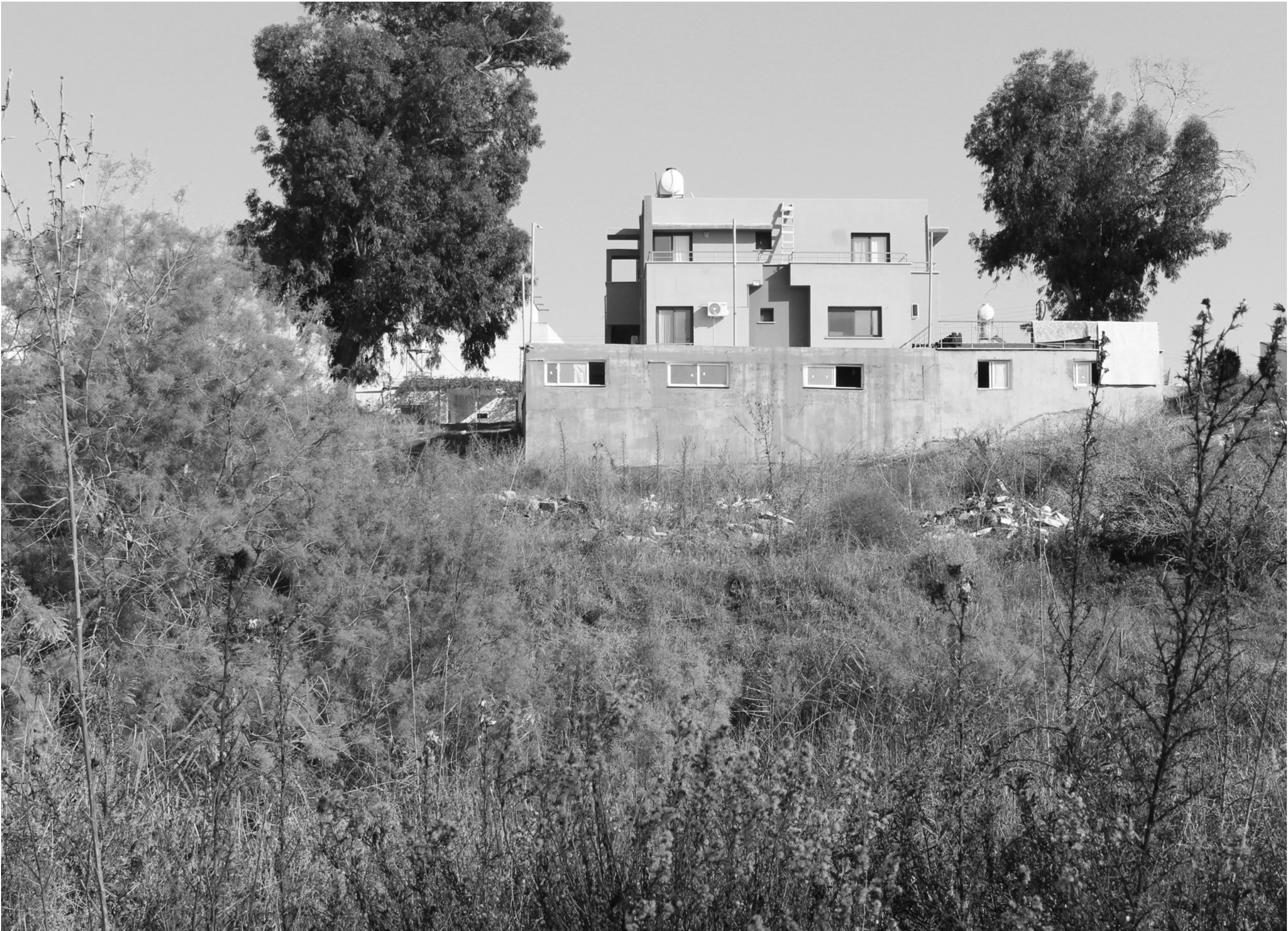
Figure 4, James Taylor, Photo of illegal construction into the land of the lake, December 2024
